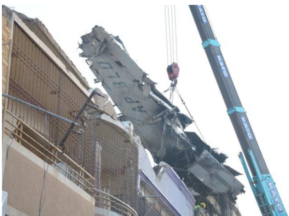
Fig 7 : Left wing being lifted from roof top
